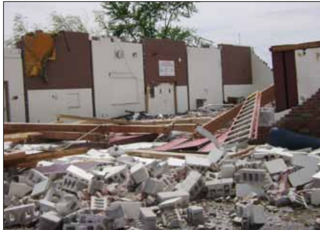
A storm on May 8 caused $500,000 worth of damage at Christ Lutheran Church and School in Jacob, Ill. The storm ripped apart the school gymnasium, and a tree fell on the roof of a classroom. Due to the damage, the school classes ended a week early this year. One member of Immanuel, Murphysboro, was killed by the storm when a tree fell through his house.
